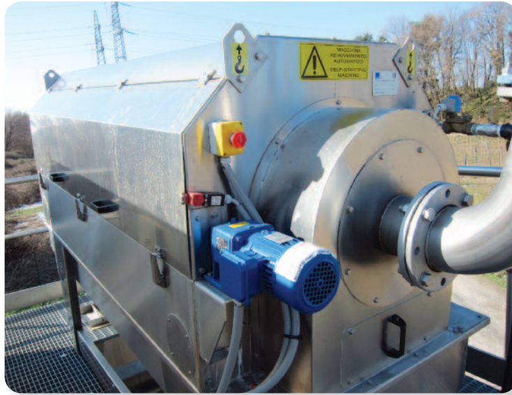
A RotoDrum Screen Pre-treating Wastewater at an MBR Installation.
