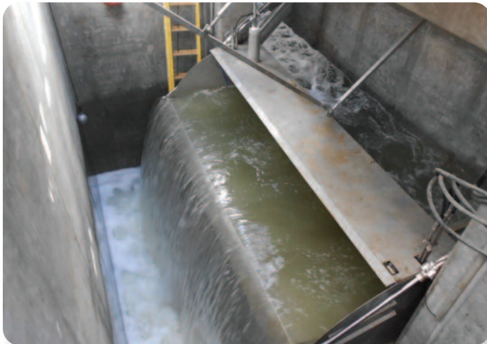
Installation of an RSW-K Weir Gate CSO screen
