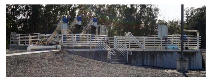
The WRF is designed to treat a buildout flow rate of 2.5 MGD at average dry weather flow conditions and 5.0 MGD at peak wet weather flow conditions. The WRF process train includes an emergency overflow basin, headworks, anoxic basins, aeration tanks with membranes, metering, and disinfection. In order to meet the projected buildout demands, the City will need to reuse 100 percent of its treated water during peak demand in the summer months.
